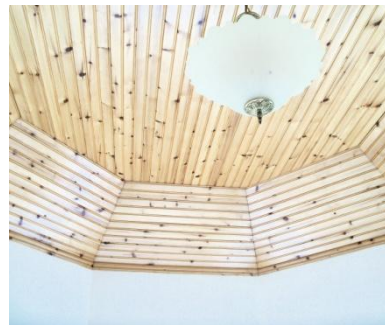
Sun Room Ceiling
